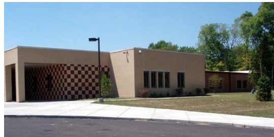
Westbrooke Village Elementary School
